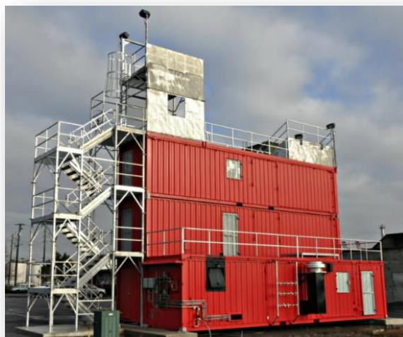
Live-Fire Training Prop – Training Center
